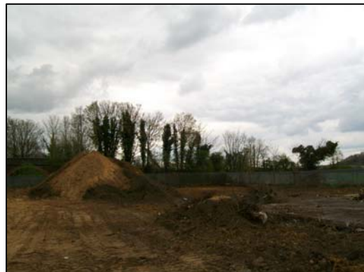
View towards northern & north-eastern boundary
